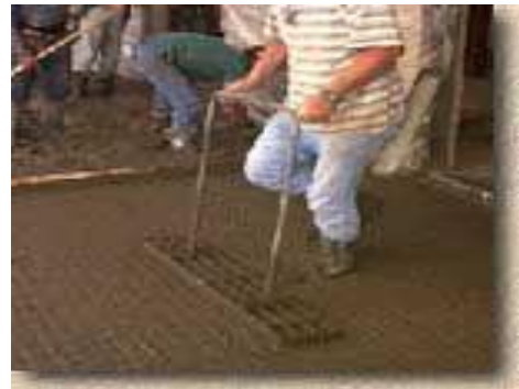
Levelling out the concrete
